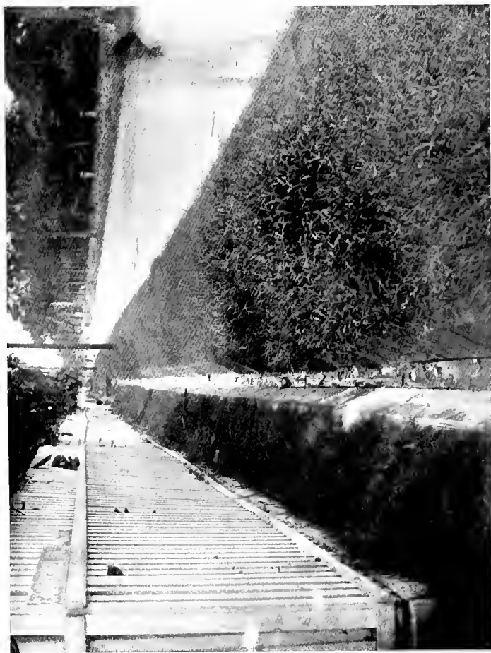
FIG. 30.—SMALL ROADSIDE CONCRETE DRAIN, PORT OF SPAIN.
